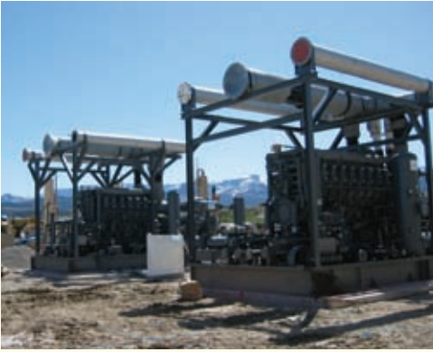
The Hunter Mesa Station Expansion was completed in August 2011.
