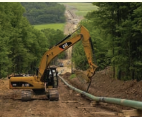
These Marcellus Pipeline projects are ongoing.
