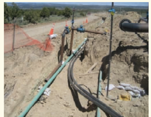
The Buck Ridge Gathering System was completed in December 2010.
