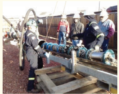
The Xcel Pipeline Modifications were completed in February 2010.
