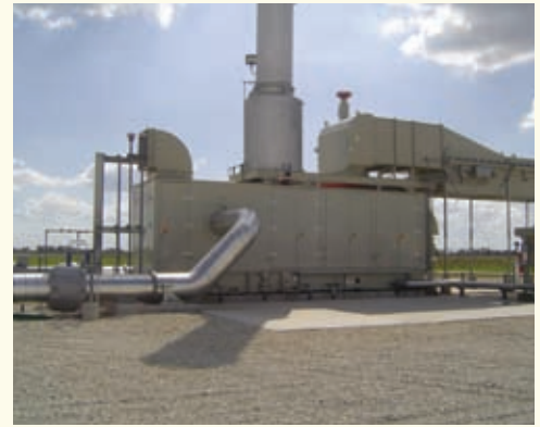
Station 430 was completed in December 2008.
