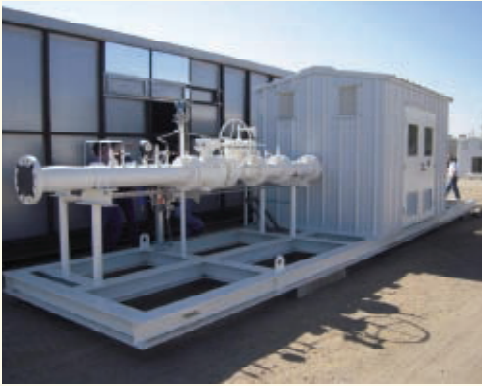
The Tiger Pipeline Expansion was completed in February 2011.
